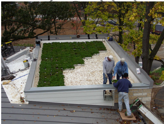
MODULAR GREEN ROOF SYSTEM INSTALLATION
