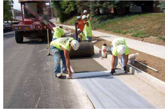
PURDUE UNIVERSITY- WEST LAFAYETTE IN PEROUS CONCRETE DRAINAGE IMPROVEMENT
