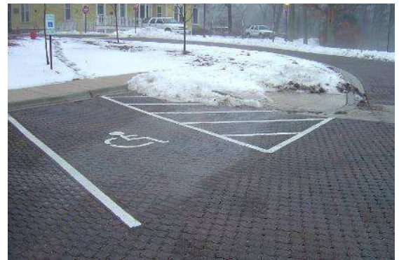
MORTON ARBORETUM- CHICAGO, IL PERMEABLE PAVER SYSTEM APPLICATION
