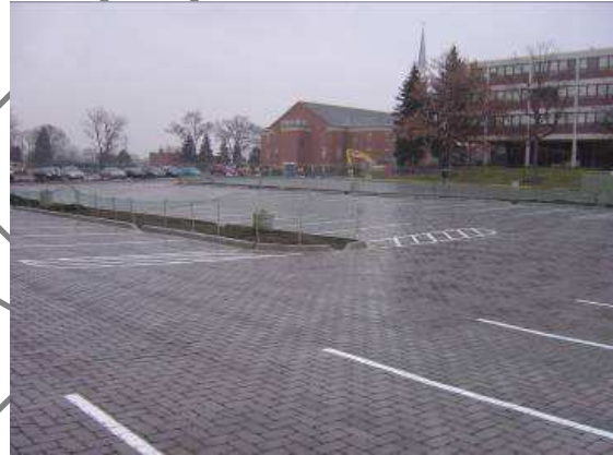
ELMHURST COLLEGE-ELMHURST ILLINOIS-PERMEABLE PAVER SYSTEM
