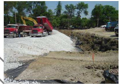
SUBBASE EXCAVATION AND CONSTRUCTION
