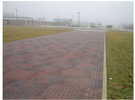
BRENTWOOD SCHOOL-PLAINFIELD, IN-PERMEABLE PAVER SYSTEM APPLICATION
