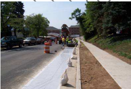
PURDUE UNIVERSITY- WEST LAFAYETTE IN PEROUS CONCRETE DRAINAGE IMPROVEMENT
