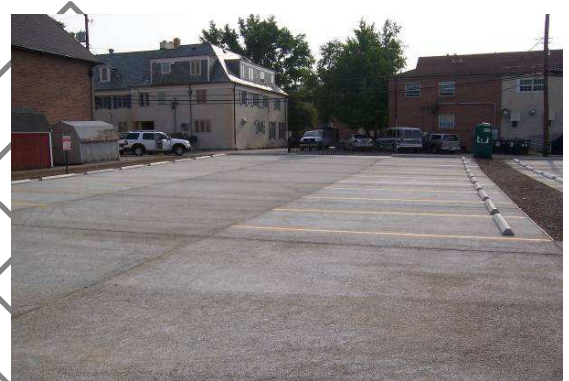
PURDUE UNIVERSITY-WEST LAFAYETTE, IN PERVIOUS CONCRETE APPLICATION
