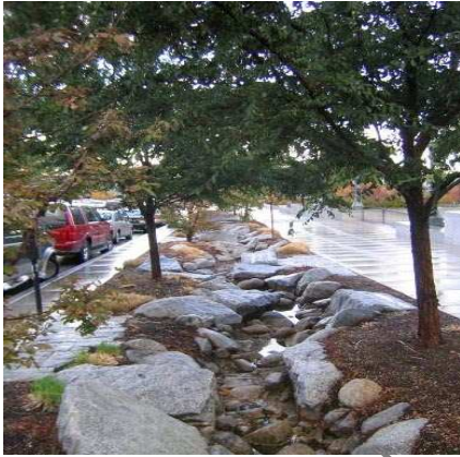
ALTERNATIVE “STREAM BED” URBAN BIORETENTION
