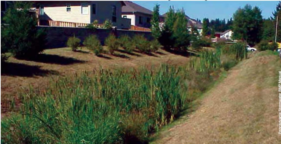
SWALE IN EASEMENT OF SUBDIVISION
