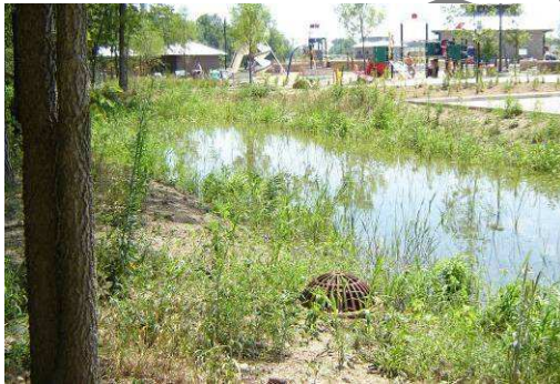
BIORETENTION POSITIVE OVERFLOW OUTLET – DILLON PARK, HAMILTON COUNTY, IN
