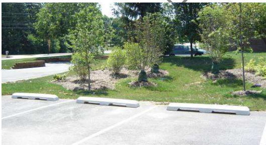
CURBLESS INLET TO BIORETENTION – INDIANAPOLIS, IN
