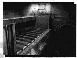
ACU-SCREEN in stormwater overflow basin.
