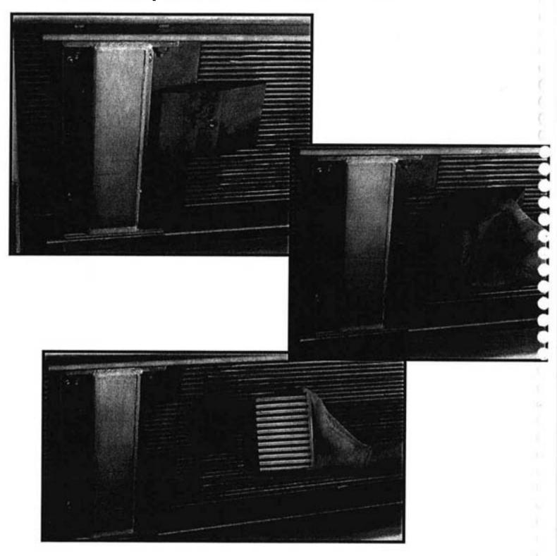
If the screen has a locking pin, place a screwdriver on the top of the pin and with the rubber mallet, gently knock the pin down and out to free the comb. Then slide the comb out of the bars.
