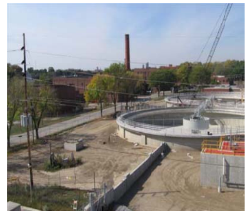
New primary treatment tanks under construction, October 2007
