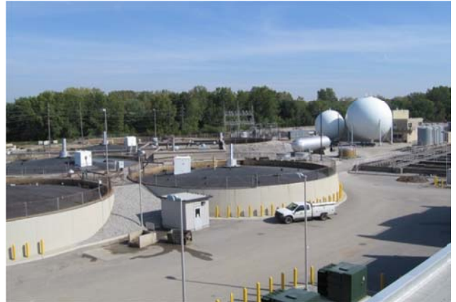
Sewage digesters produce methane gas that is collected in storage "globes" and used in the Plant
