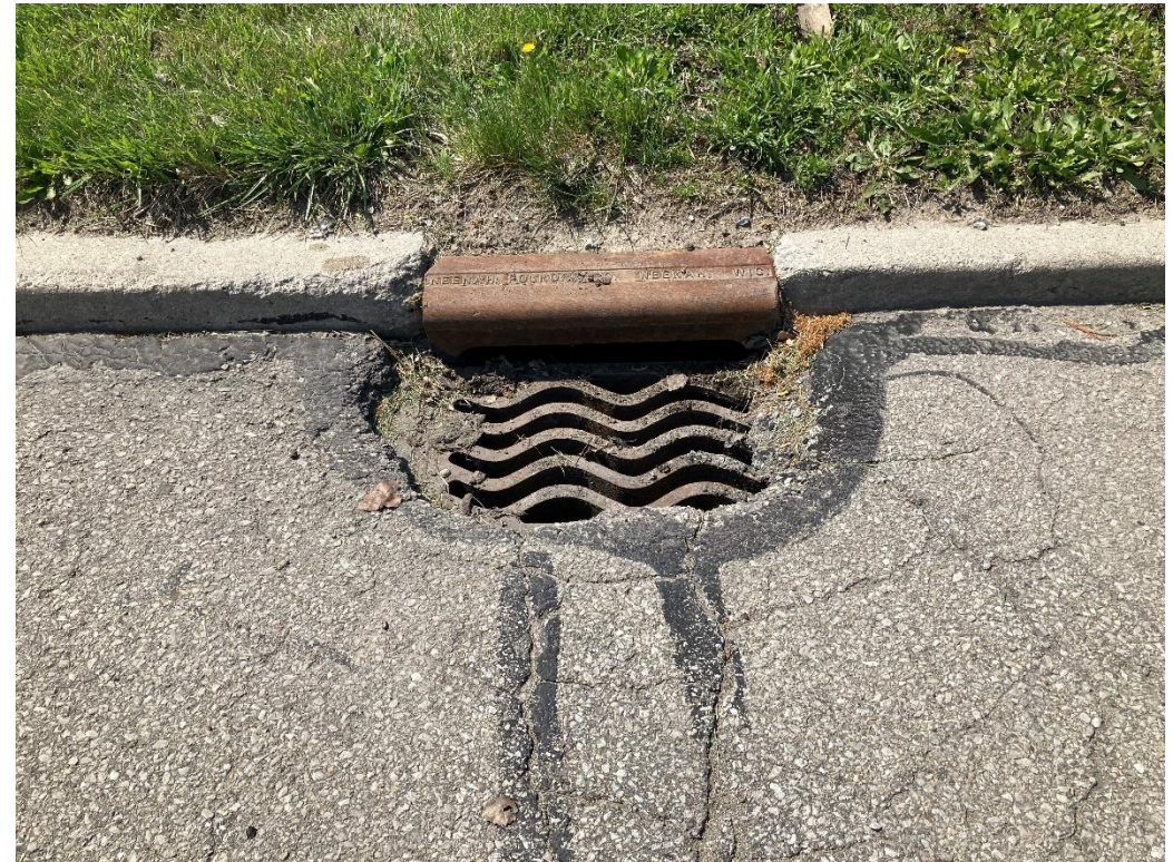
Storm Inlet After Cleaning
