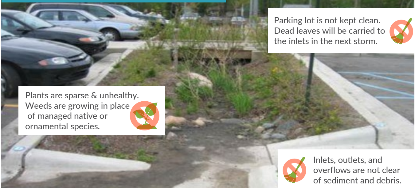
Poorly-maintained bioretention area in an asphalt parking lot
