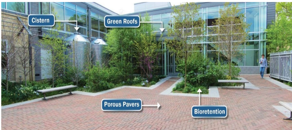
Some properties have multiple BMPs, which all require maintenance. This building has cisterns, green roofs, porous pavers, and a small bioretention area.
