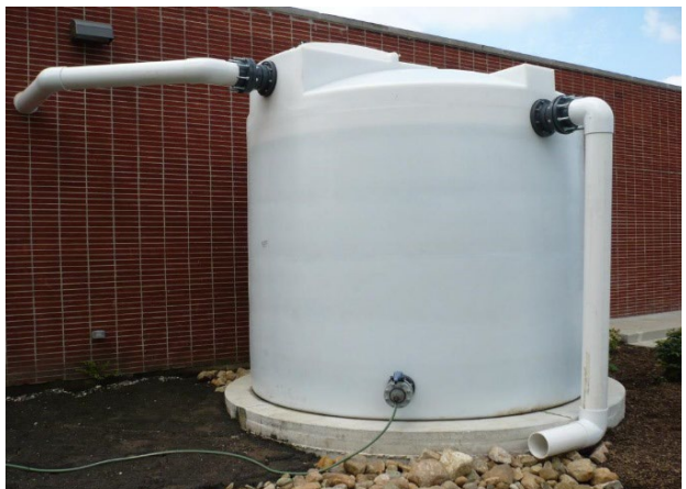
The pervious paver parking lot (left) and the cistern (right) are examples of non-vegetated BMPs.
