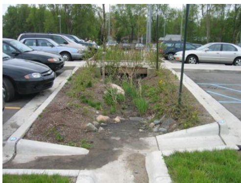
The bioretention area in this parking lot island has accumulated sediment which requires removal.
