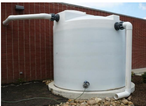
The pervious paver parking lot (left) and the cistern (right) are examples of non-vegetated BMPs.
