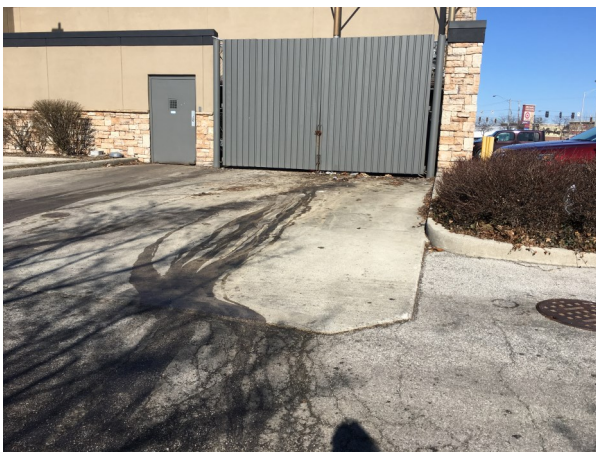
Leaking dumpster area
