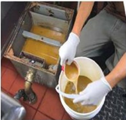
Employee cleaning grease trap
