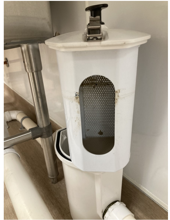
Side view of removed basket
