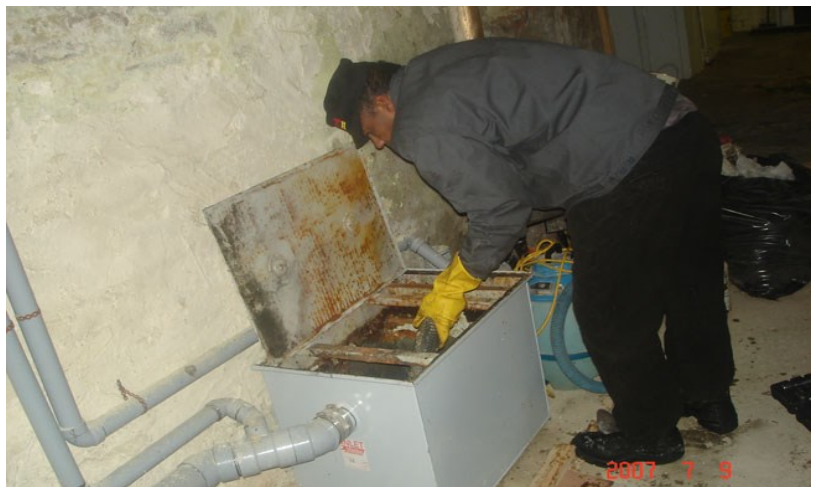
Employee cleaning grease trap with shop-vac
