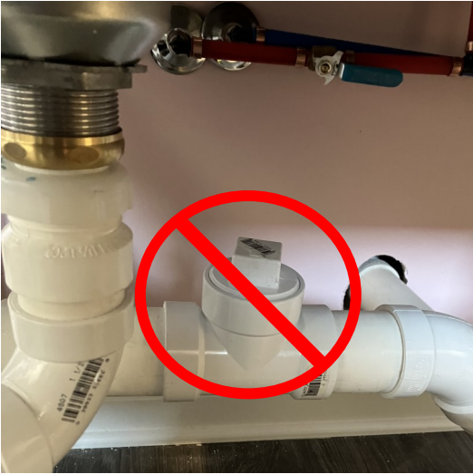
Cleanouts cannot be used as sampling ports
