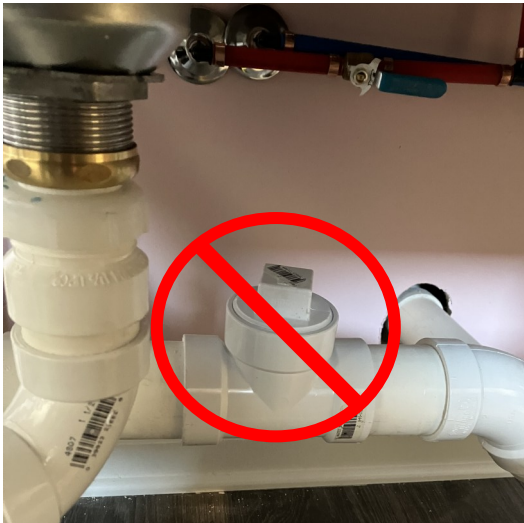
Cleanouts cannot be used as sampling ports
