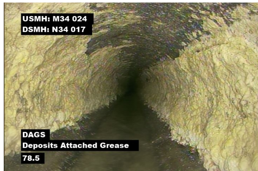
Fats, oils, and grease build-up in sewer main line near Glenbrook mall
